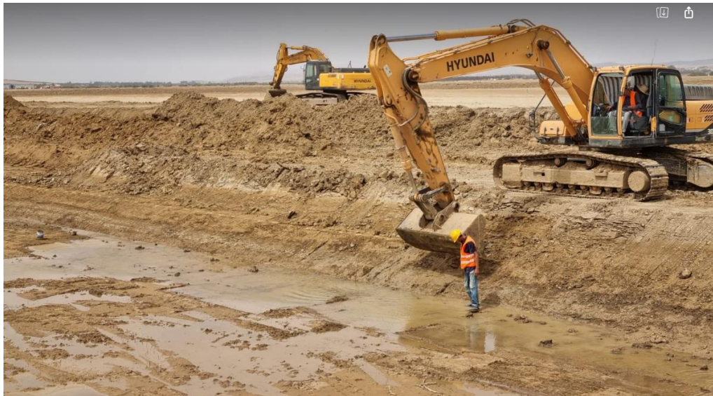
Cleaning of waterways, Medjerda flood protection project (Source: general direction of dams and large hydraulic works))
