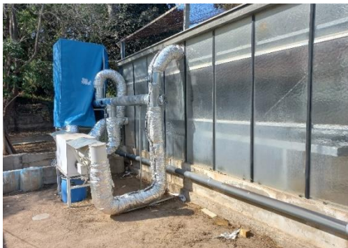
The experimental greenhouse of the national institute of research in rural engineering water and forests with the new device of thermal dissipation next to the absorption system
